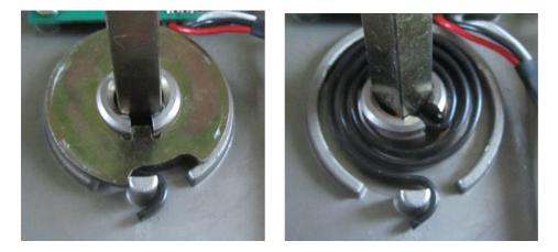
If you want the handle on the right hand side (seen from the outer door side), place the spring and the metal plate like below.
